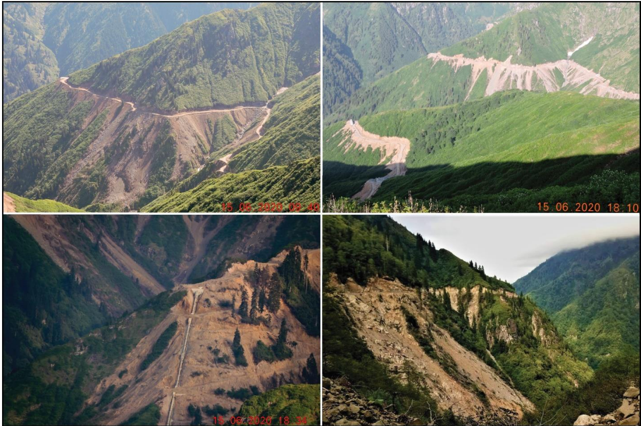
Figure 5. Photos showing the mass movements on hillslopes associated with road constructions of HEPP . The photos were taken on 15 th June 2020 (Photographs courtesy of Hasan Sıtkı Özkazanç).
