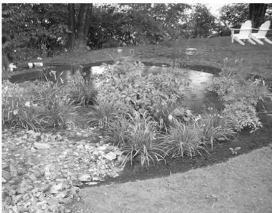
Rain gardens or bioretention svstems hold water during storms and release it slowly.
