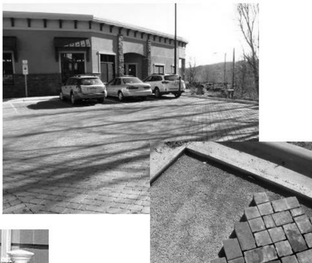
Permeable pavement allows water to soak through it rather than running off of it.
